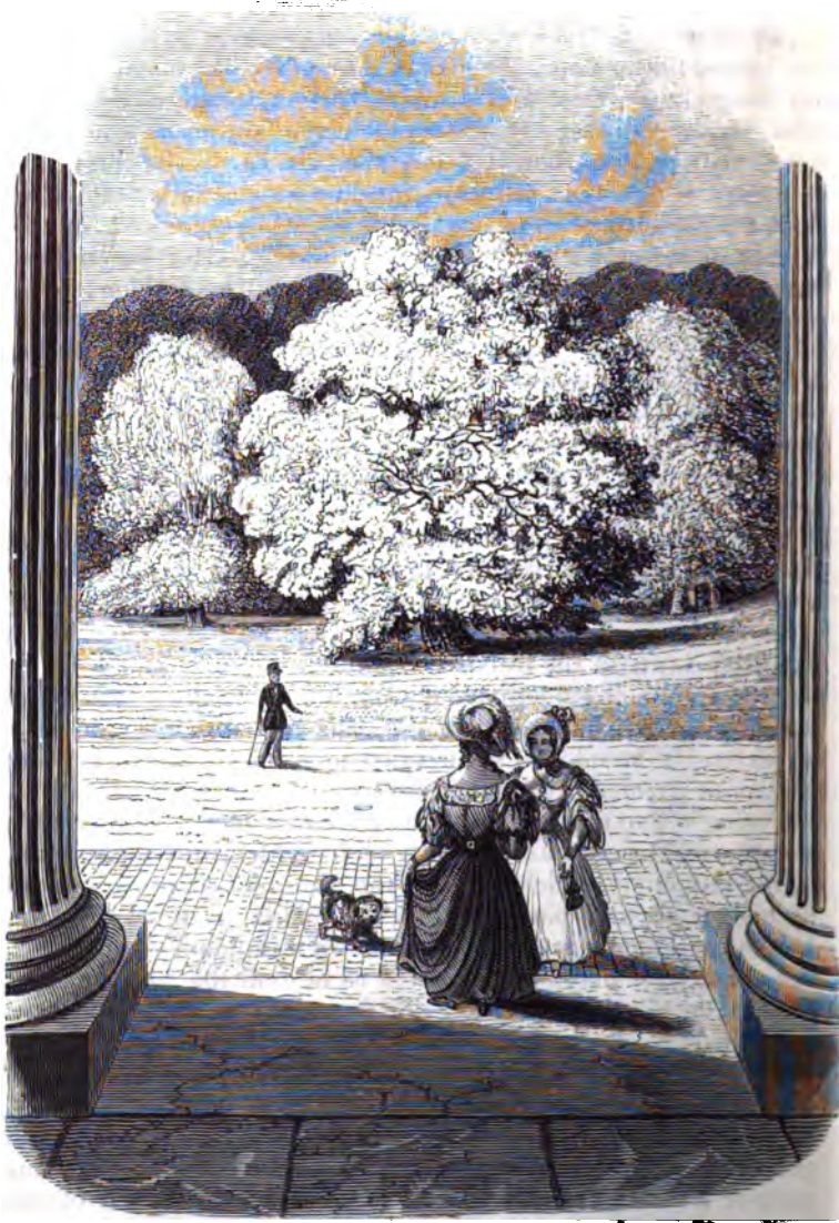
View from the Entrance Portico at Kenwood.
